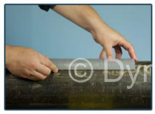
To install, confirm that the DynaGard fits snugly onto the pipe to be protected
