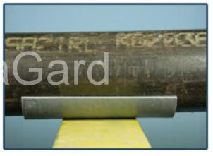
With the DynaGard in place, lower the pipe back on to the support.
